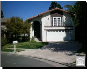
*Bank owned. Really rough, but bank is doing some repairs.
